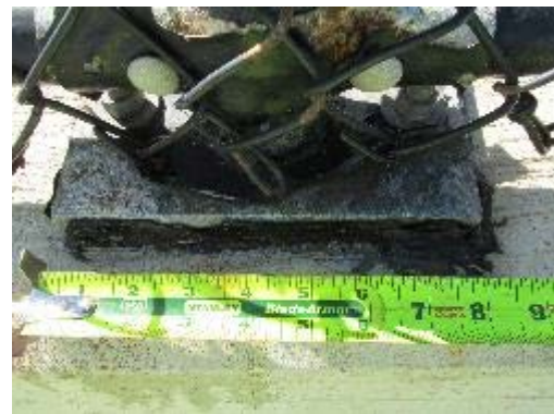
Caulk around fence attachment plate
