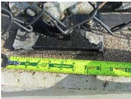
Caulk around fence attachment plate
