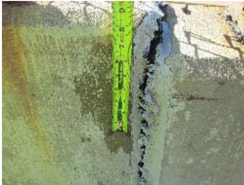
Caulk in abutment joint
