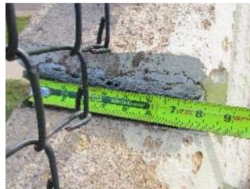
Caulk in abutment joint
