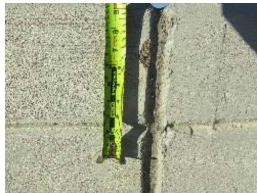
Caulk in parapet expansion joint
