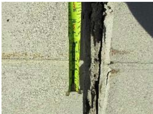
Caulk in abutment joint
