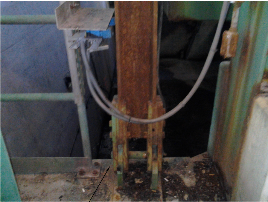
CLEAN AND PAINT REAR LOCK AT EACH LOCATION (4 TOTAL)
