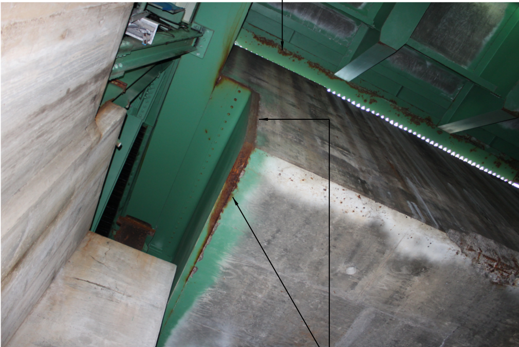
CLEAN AND PAINT END AND UNDERSIDE EDGES OF COUNTERWEIGHT
