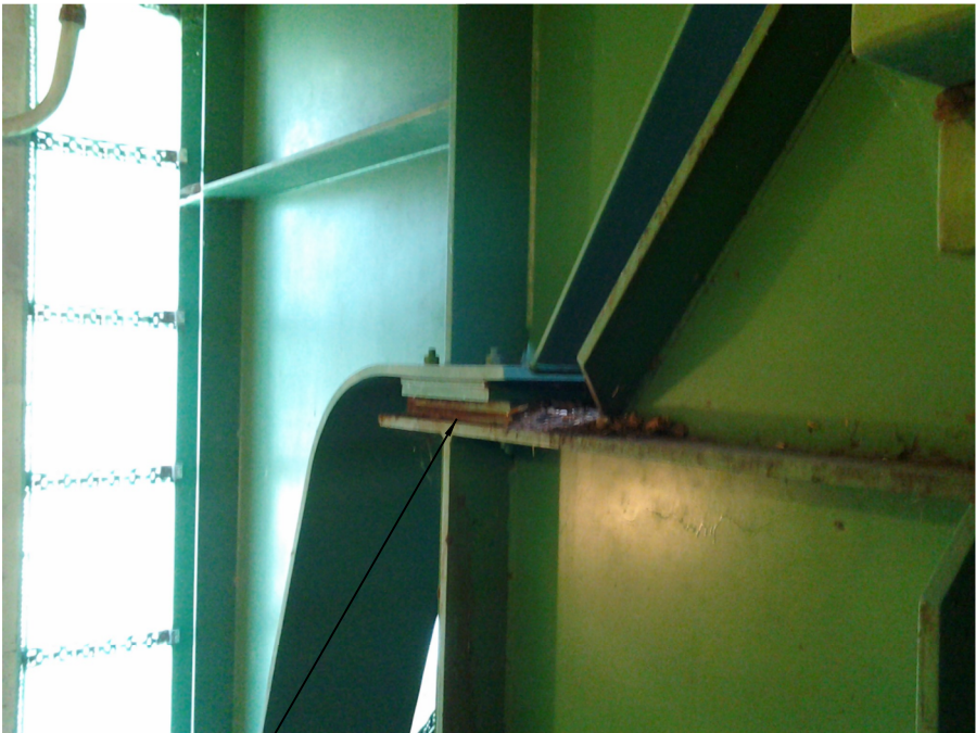
CLEAN AND PAINT LIVE LOAD UPLIFT SUPPORT PLATES/SHIMS
