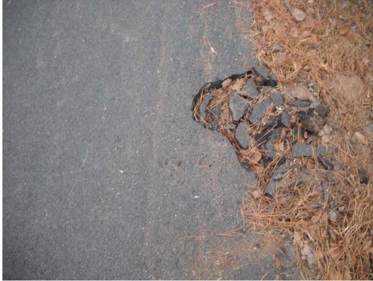
Road Damage from Logging Truck Outrigger
