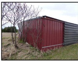
View of southern shed
