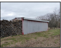
View of southern shed
