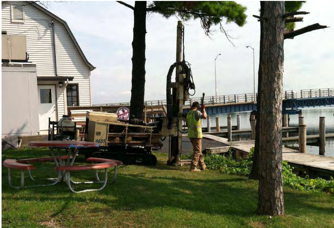
Site #8: Location of boring B-8-3 near former coal storage area.
