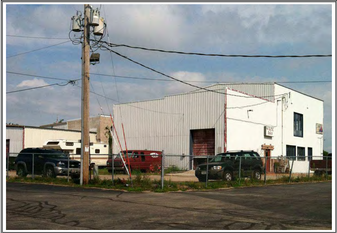
Site #5: View of southeast corner of property from alley; location of boring B-5-3.
