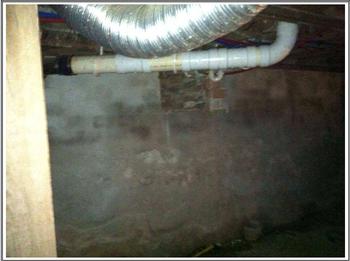
Site #12: Interior view (basement) of former coal chute area.
