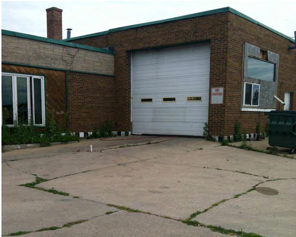
Site #11: Location of boring B-11-1 (PVC riser).
