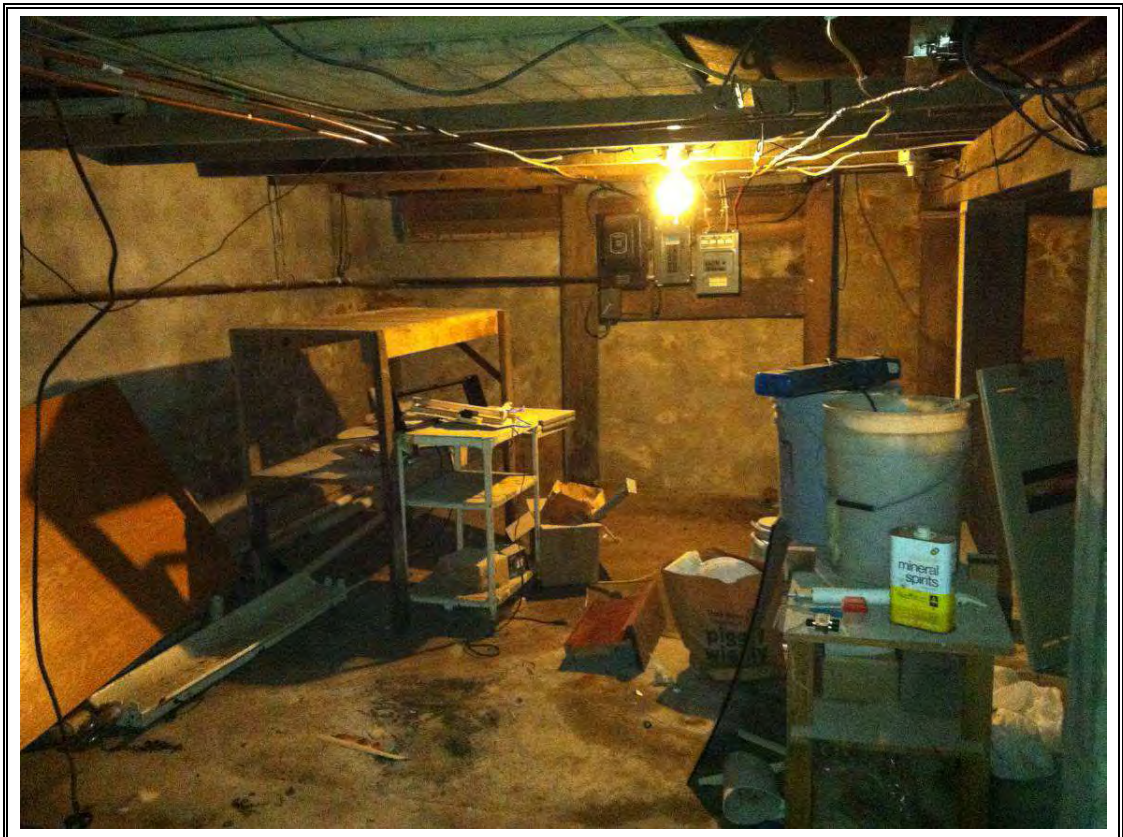
Site #12: Interior view of basement
