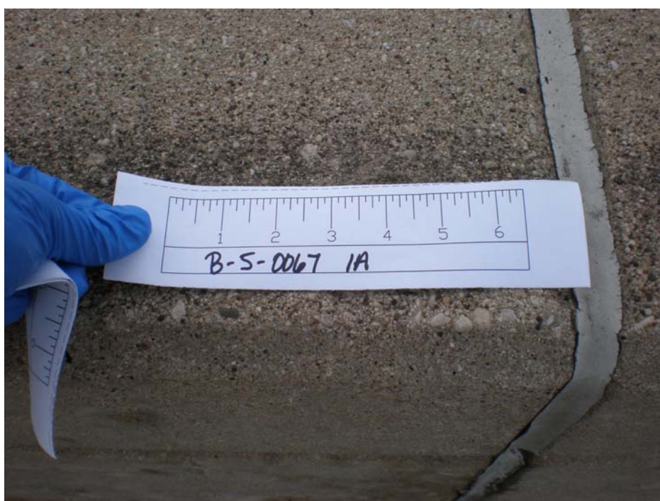
Gray caulk located on the parapet walls of Structure B-05-0067.
