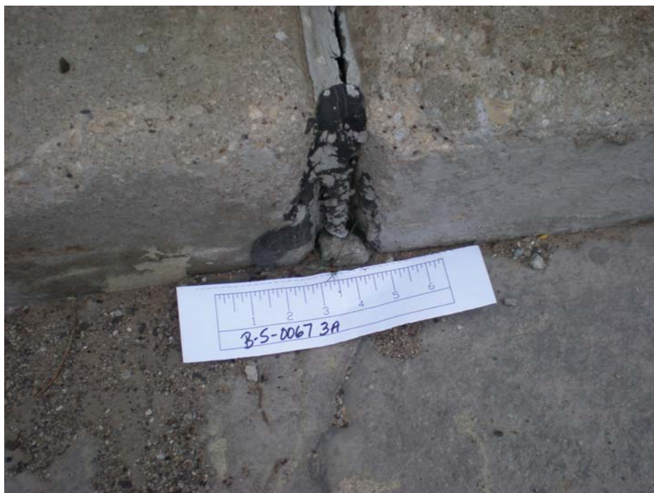
Black tar located on the deck of Structure B-05-0067.
