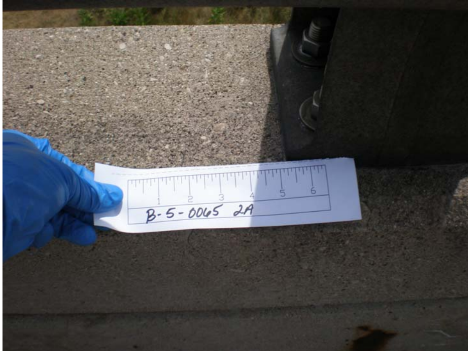
Guard rail base plate gasket located on the parapet wall of Structure B-05-0065.
