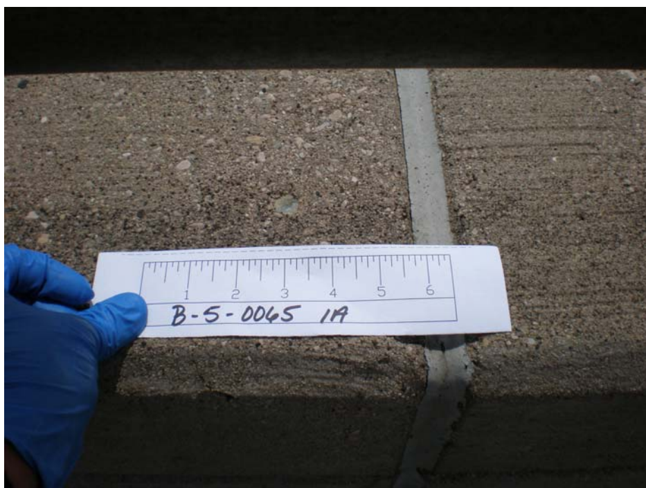
Gray parapet wall caulk located on Structure B-05-0065.
