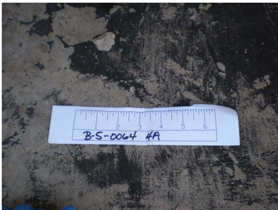
Black paint/tar located on the underside of Structure B-05-0064.
