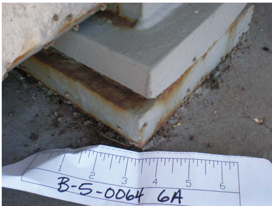
Brown fibrous gasket located beneath bearing pad under structure B-05-0064.
