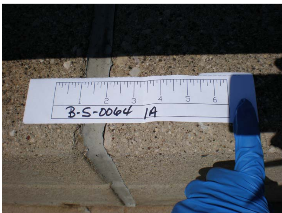
Gray caulk located on the parapet wall joint of Structure B-05-0064.
