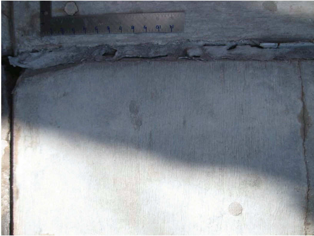
Caulk in abutment expansion joint
