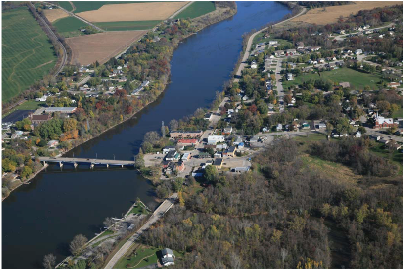
This photo shows the currently existing bridge. Left side of bridge is west and right side is east.
