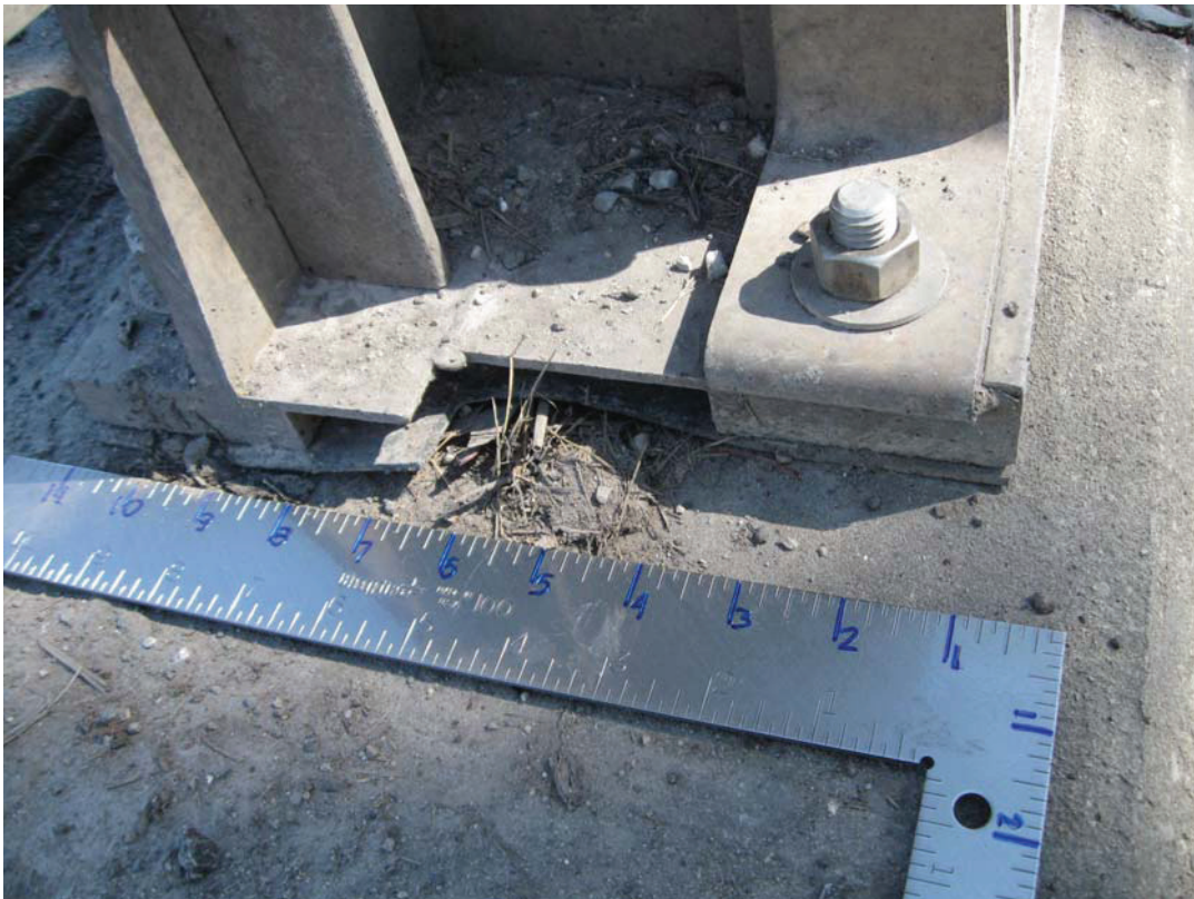
Black rubber mat under guardrail attachment is not assumed to be asbestos-containing therefore no samples were collected.
