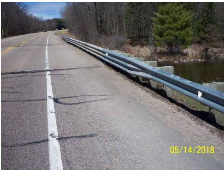
Photo 1.4 Thrie beam transition at the Crystal River Bridge
