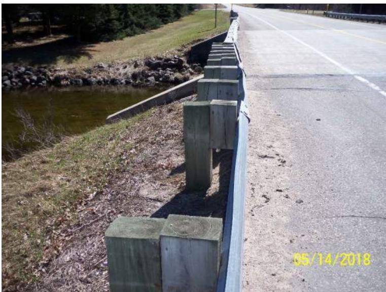
Photo 1.8 Inward deflection the guardrail off the structure railing at the northeast corner
