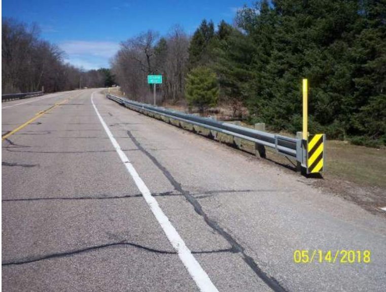
Photo 1.5 Straight taper from thrie beam transition to EAT (SE Corner)
