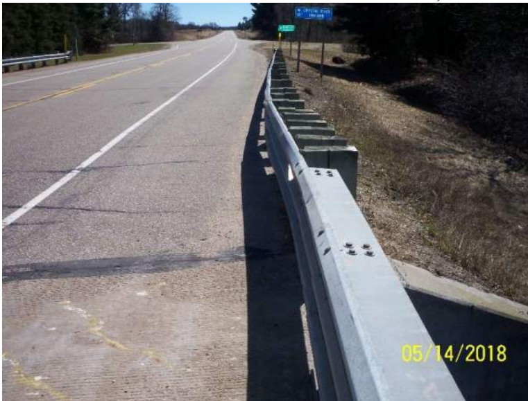
Photo 1.7 Inward deflection the guardrail off the structure railing at the southwest corner
