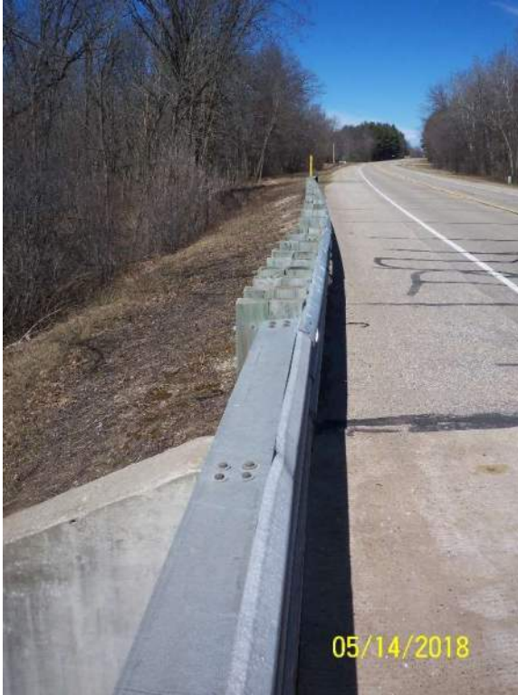
Photo 1.9 Inward deflection the guardrail off the structure railing at the northwest corner
