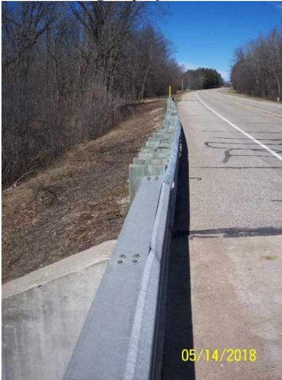
Photo 1.6 Straight taper from thrie beam transition to EAT (NW Corner)
