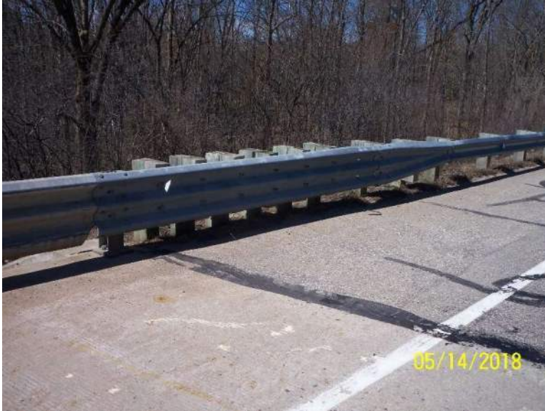
Photo 1.3 Thrie beam transition at the Crystal River Bridge
