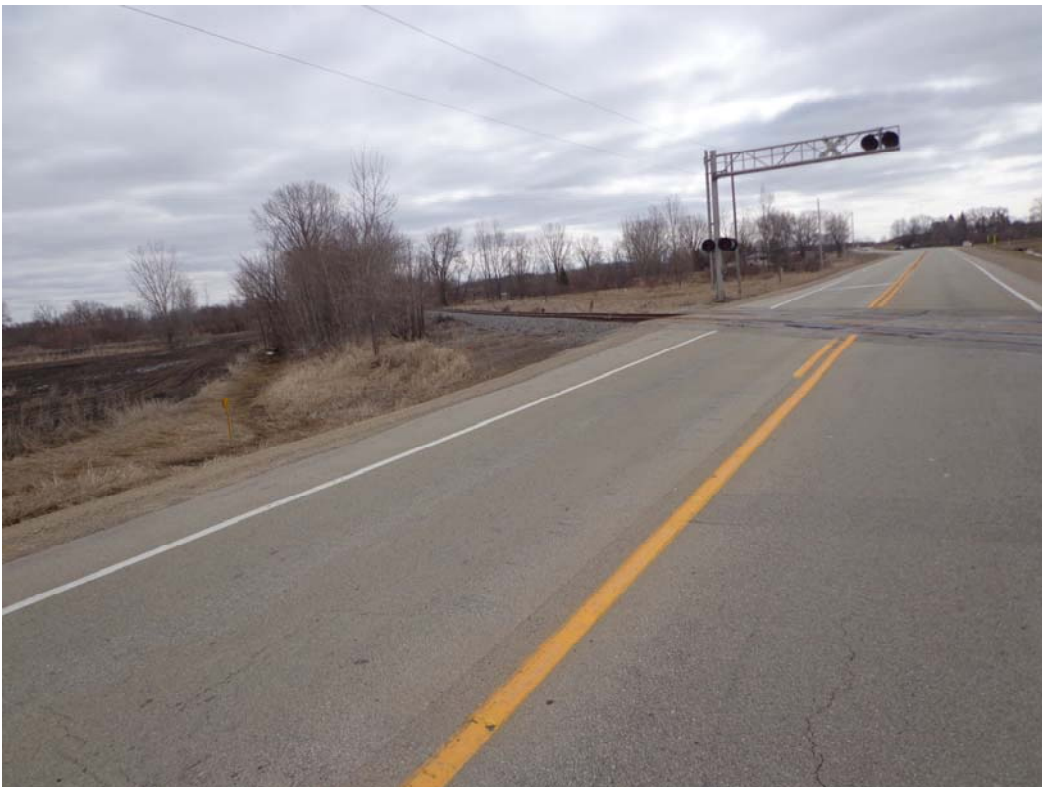
Photo #6 At Stop Clearing Sight Distance Left (North)
