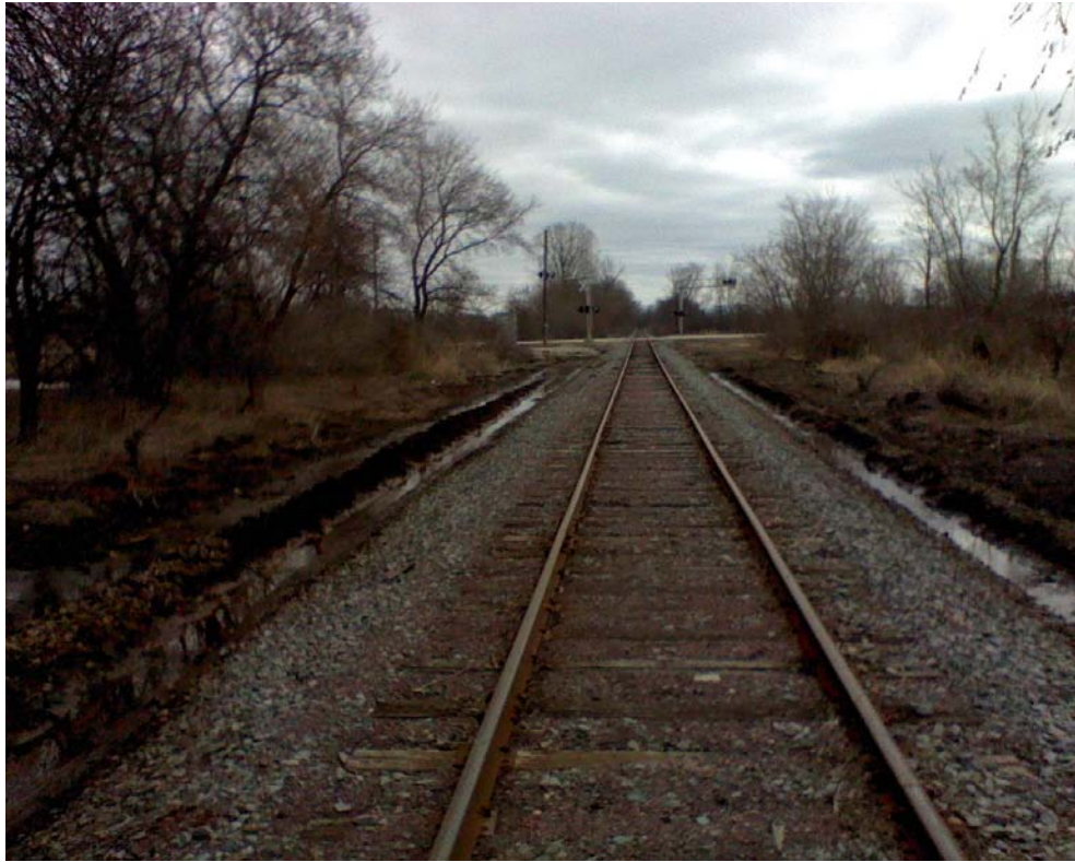
CENTERLINE OF RAIL LOOKING NORTHEASTERLY
