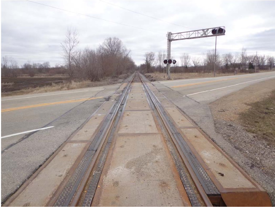
Photo #9 At Crossing CL Down Track Left (North)
