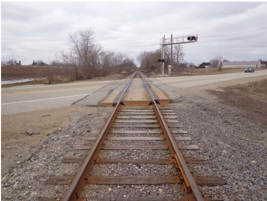
Photo #10 At Crossing CL Down Track Right (South)
