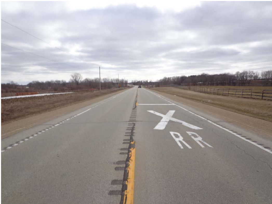
Photo #2 At SSD Entire Crossing
