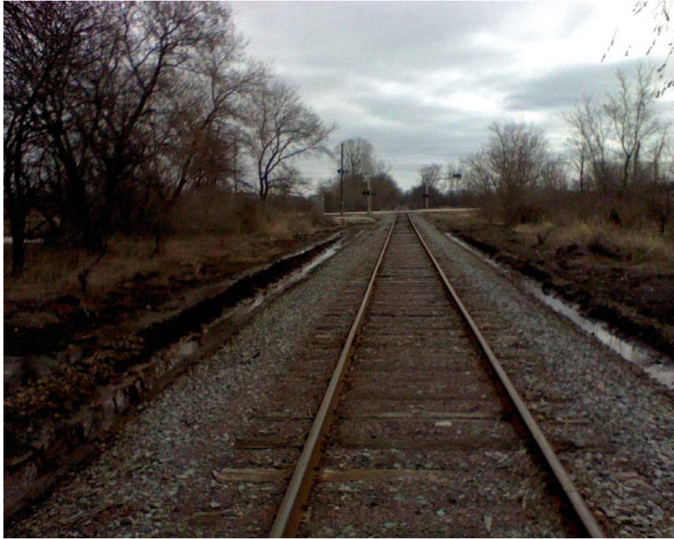
CENTERLINE OF RAIL LOOKING NORTHEASTERLY
