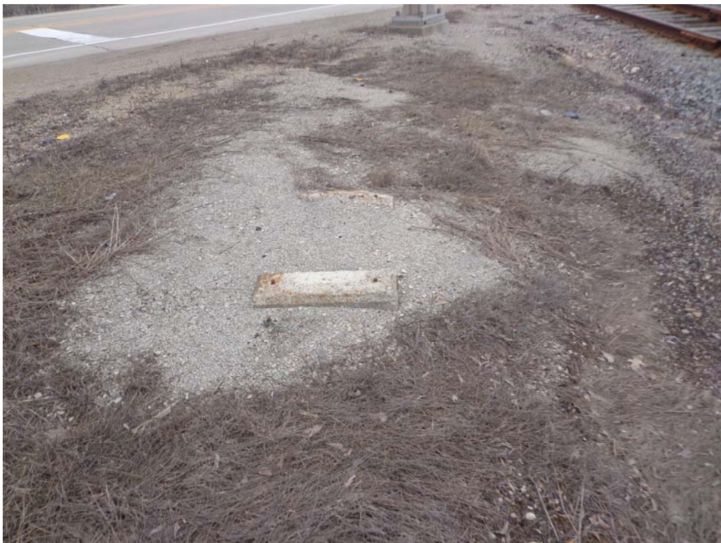
Photo #12 Other Features – Old Signal/Cabinet Base
