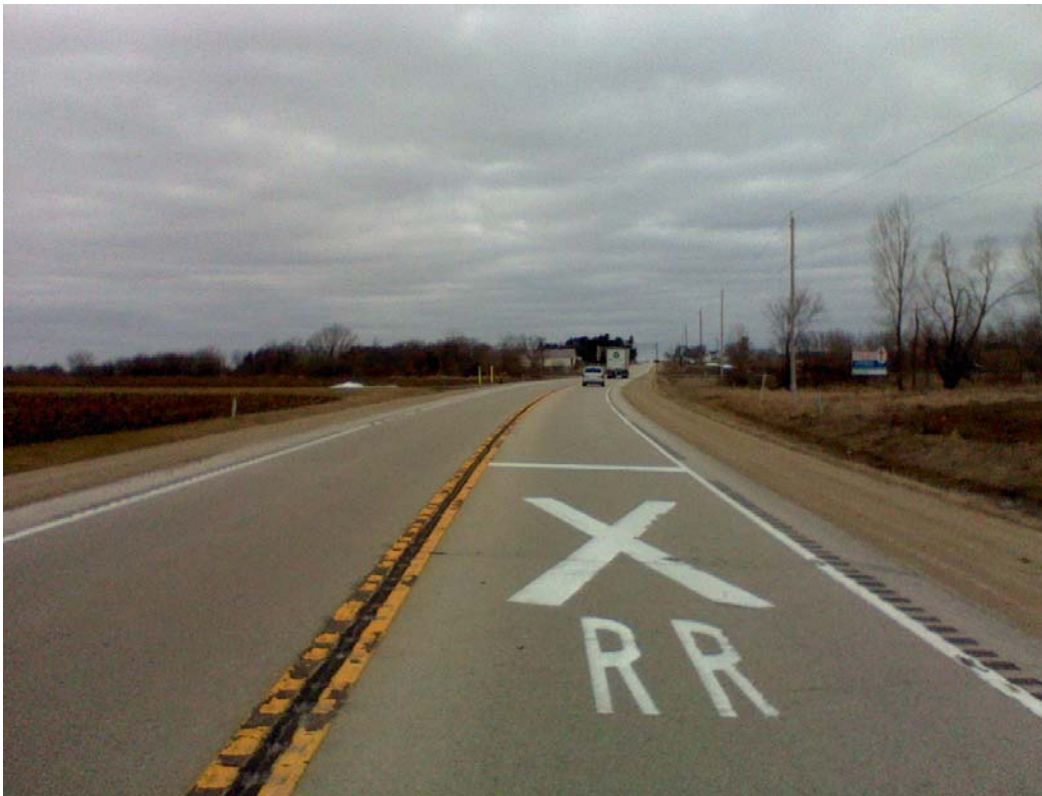
Photo #18 At SSD Entire Crossing
