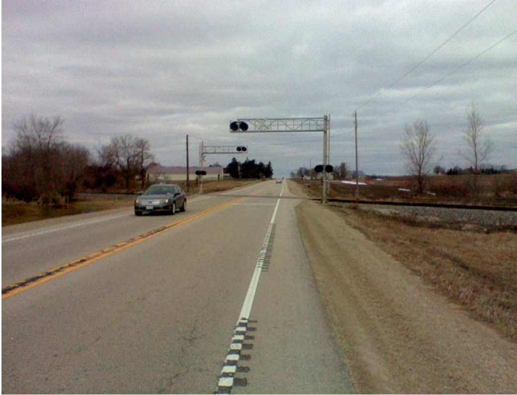
Photo #15 Approaching Stop Warning Devices
