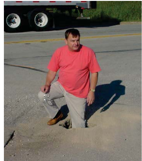
Figure 2: Improper SUE Restoration
