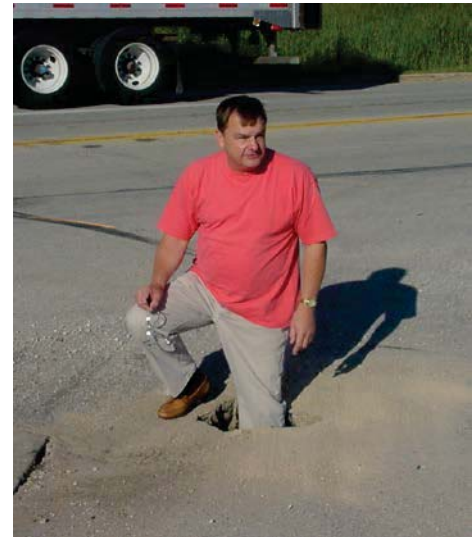
Figure 2: Improper SUE Restoration
