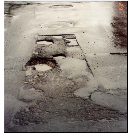
Figure 4: Both patches improperly backfilled and compacted and not patched to the nearest joint or seam.
