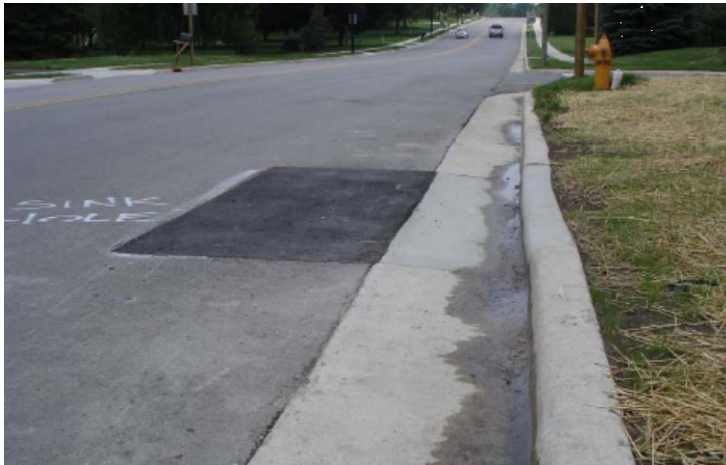
Figure 4: Both patches improperly backfilled and compacted and not patched to the nearest joint or seam.
