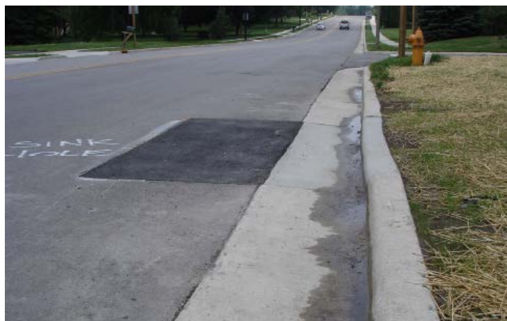
Figure 4: Both patches improperly backfilled/compacted, and not patched to nearest joint or seam
