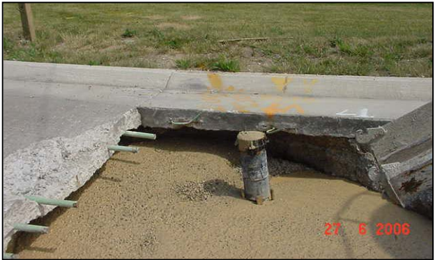
Figure 2: Concrete pavement repair without sawcut. Note top of pavement edge and missing dowel bar. In lower picture, dowel bars in gutter are bent and not ready to accept slurry.
