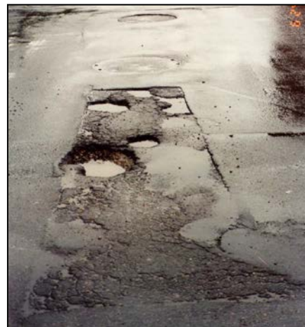
Figure 4: Both patches improperly backfilled/compacted, and not patched to nearest joint or seam
