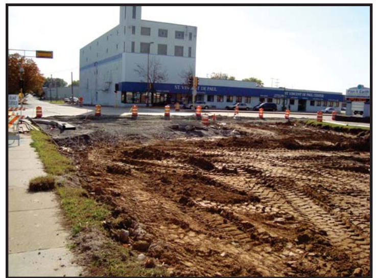
ARNOLD STREET LOOKING EAST (UNDER CONSTRUCTION AT TIME OF PHOTO)
