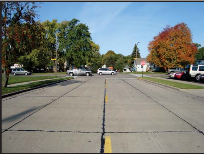
FRANKLIN STREET LOOKING WEST
