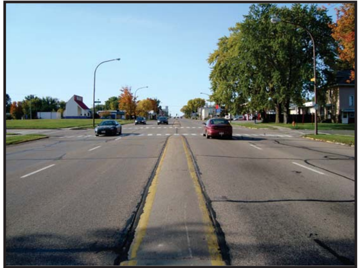
STH 97 LOOKING SOUTH
