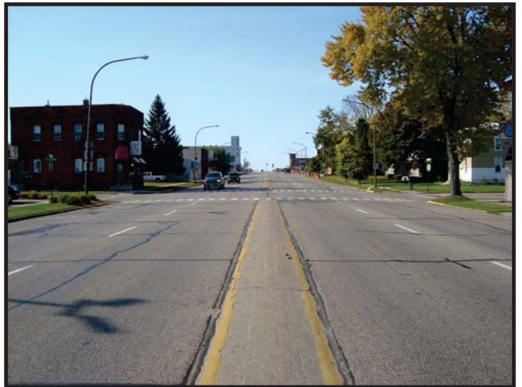
STH 97 LOOKING SOUTH
