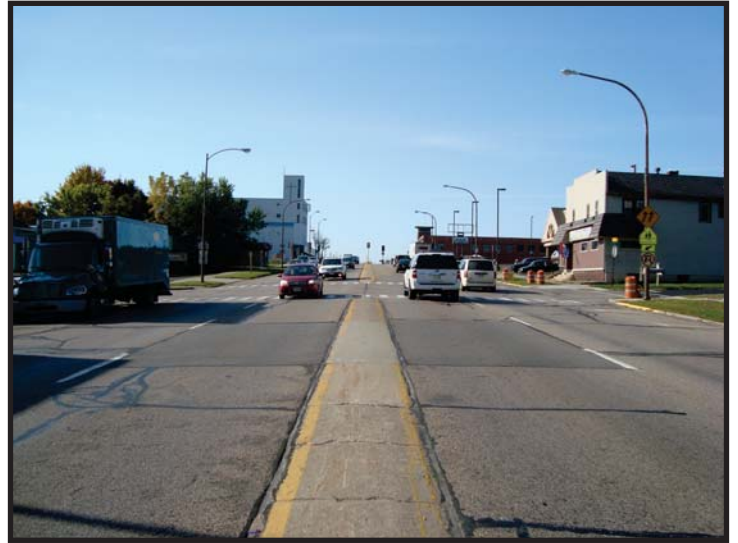
STH 97 LOOKING SOUTH
