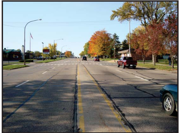
STH 97 LOOKING SOUTH
