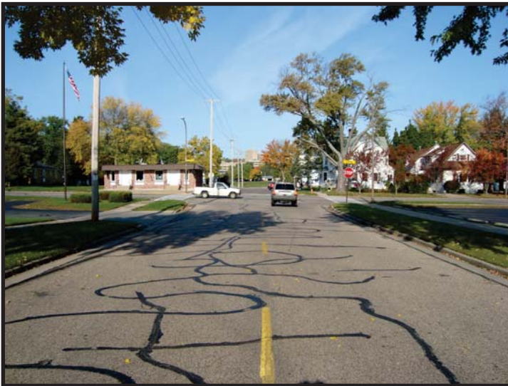
GRANT STREET LOOKING WEST
