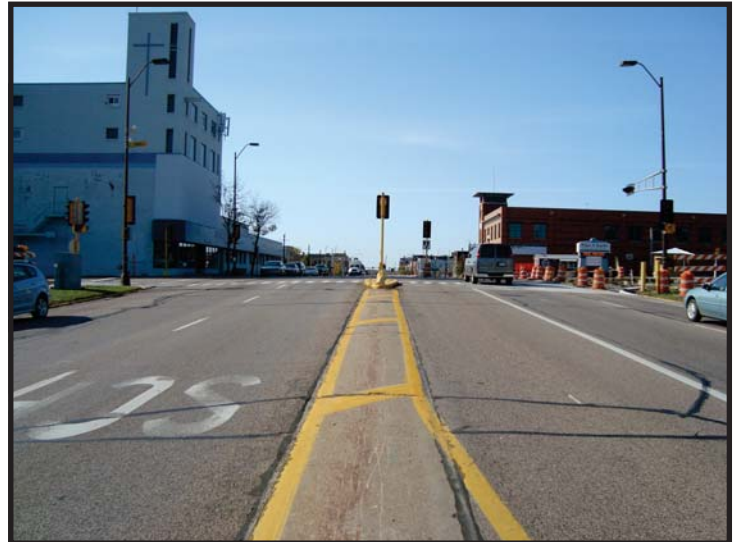
STH 97 LOOKING SOUTH
