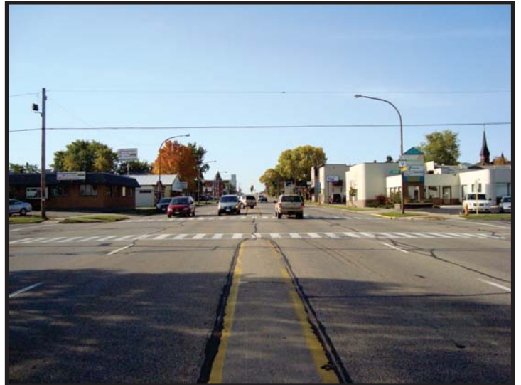
STH 97 LOOKING SOUTH
