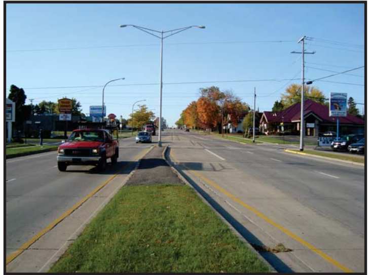
STH 97 LOOKING SOUTH
