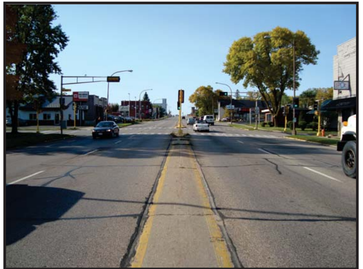
STH 97 LOOKING SOUTH
