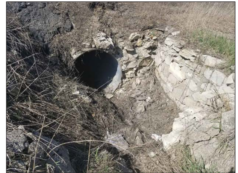
EXISTING PIPE AND STONE HEADWALL
