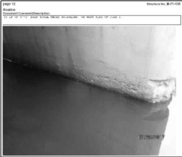
PHOTO B (6"-12" DEEP SPALL - WEST SIDE OF PIER 1)
