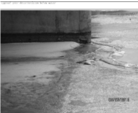
PIER (NOTE DETERIORATION BELOW WATERLINE)
