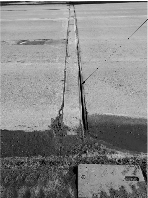
NORTH ABUTMENT (STRIP SEAL)
