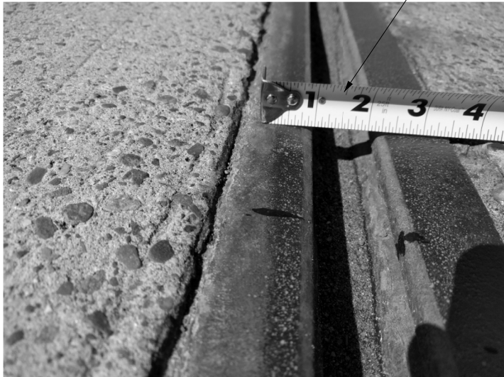
NORTH ABUT. (STRIP SEAL GAP MEASUREMENT)
