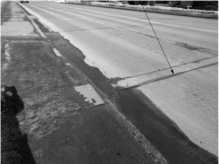
NORTH ABUTMENT (STRIP SEAL AT SIDEWALK/GUTTER)
