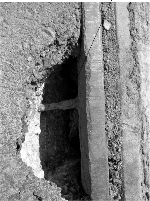
NORTH ABUTMENT (STRIP SEAL AT C)
