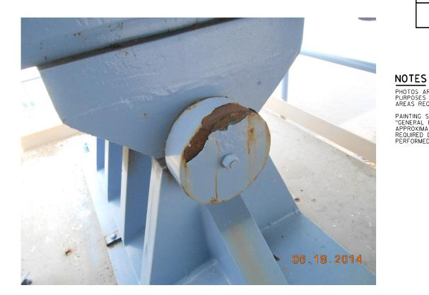
TYPICAL ISOLATED CORROSION ON BEARING AT PIER 5
