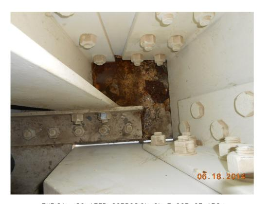
TYPICAL ISOLATED CORROSION ON FLOOR OF ARCH INSIDE TIE GIRDER IN SPAN 5
