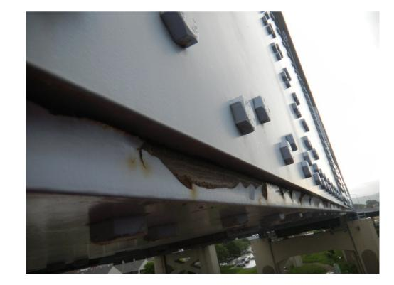
TYPICAL ISOLATED CORROSION ON ARCH TIE GIRDER IN SPAN 5
