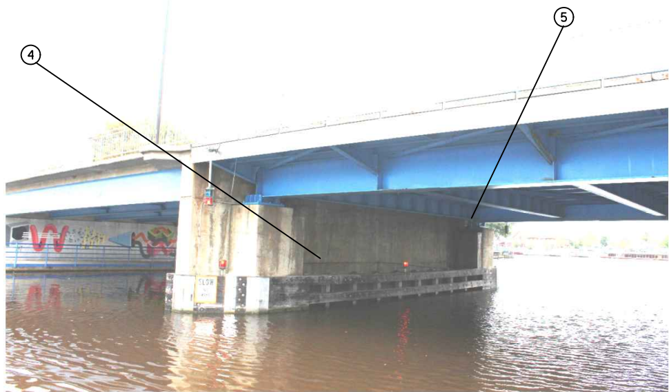
PIER 2 NAVIGATION LIGHTS AND CONDUIT
