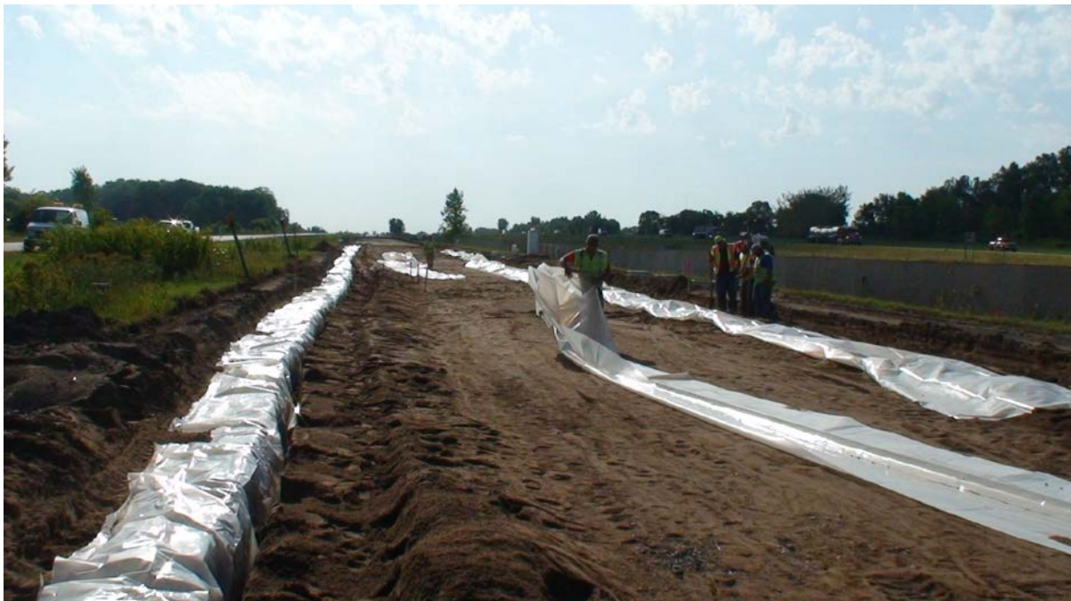
Figure 4.1. Cell 86 (sand subgrade) installing plastic edge barriers
