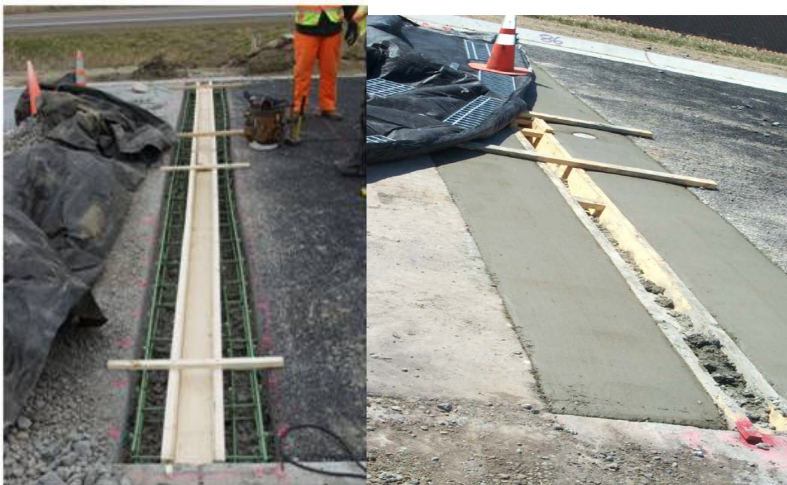
Figure 4.10. Cell-separating transverse drains
