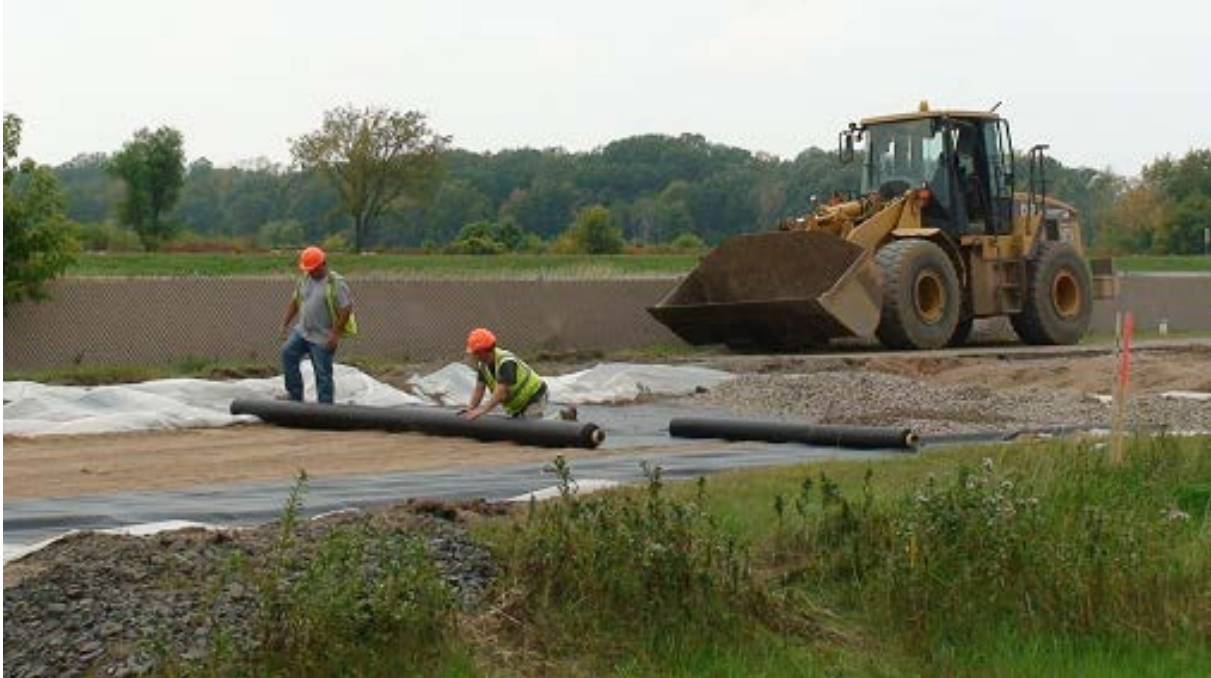
Figure 4.3. Installation of type V geotextile
