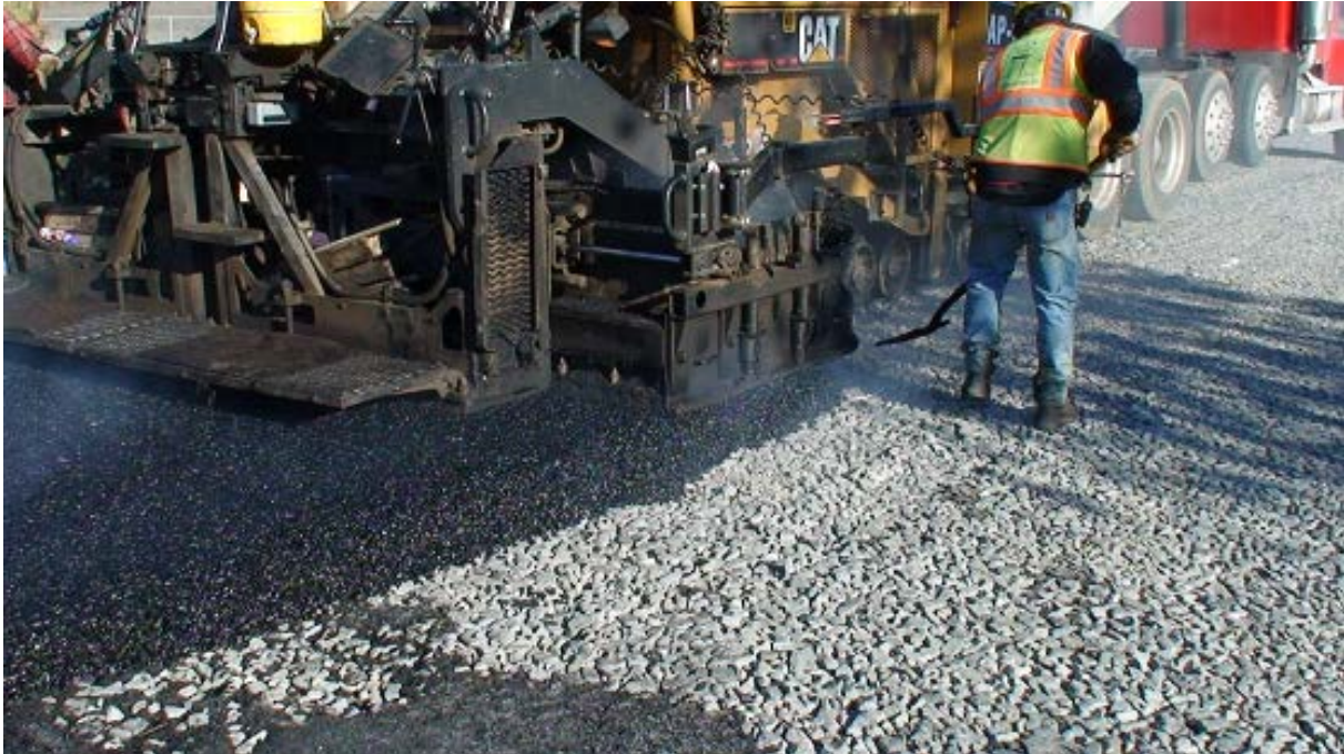
Figure 4.8. Porous asphalt paving
