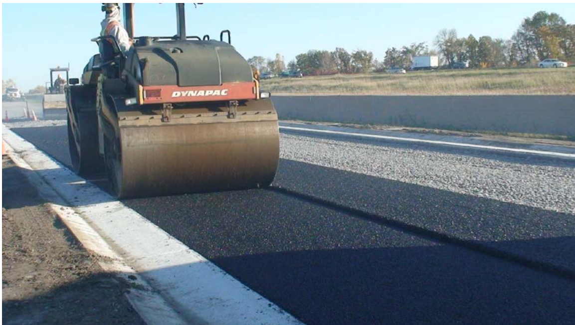
Figure 4.9. Porous asphalt rolling
