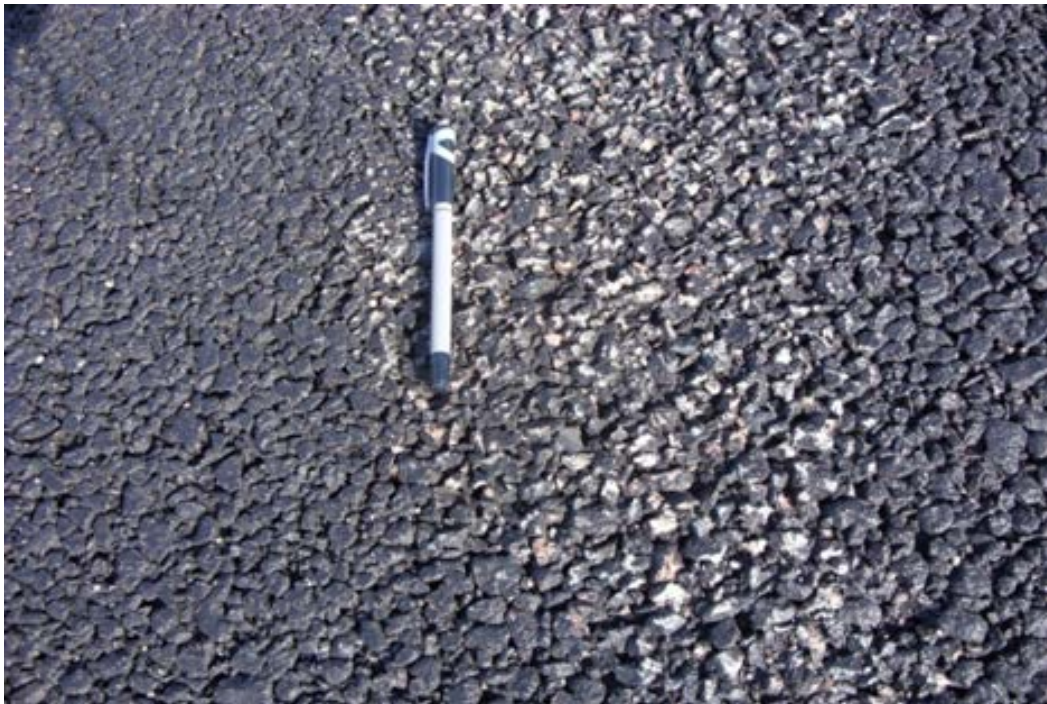
Figure 5.11. Minor snowplow scuffing, cell 86
