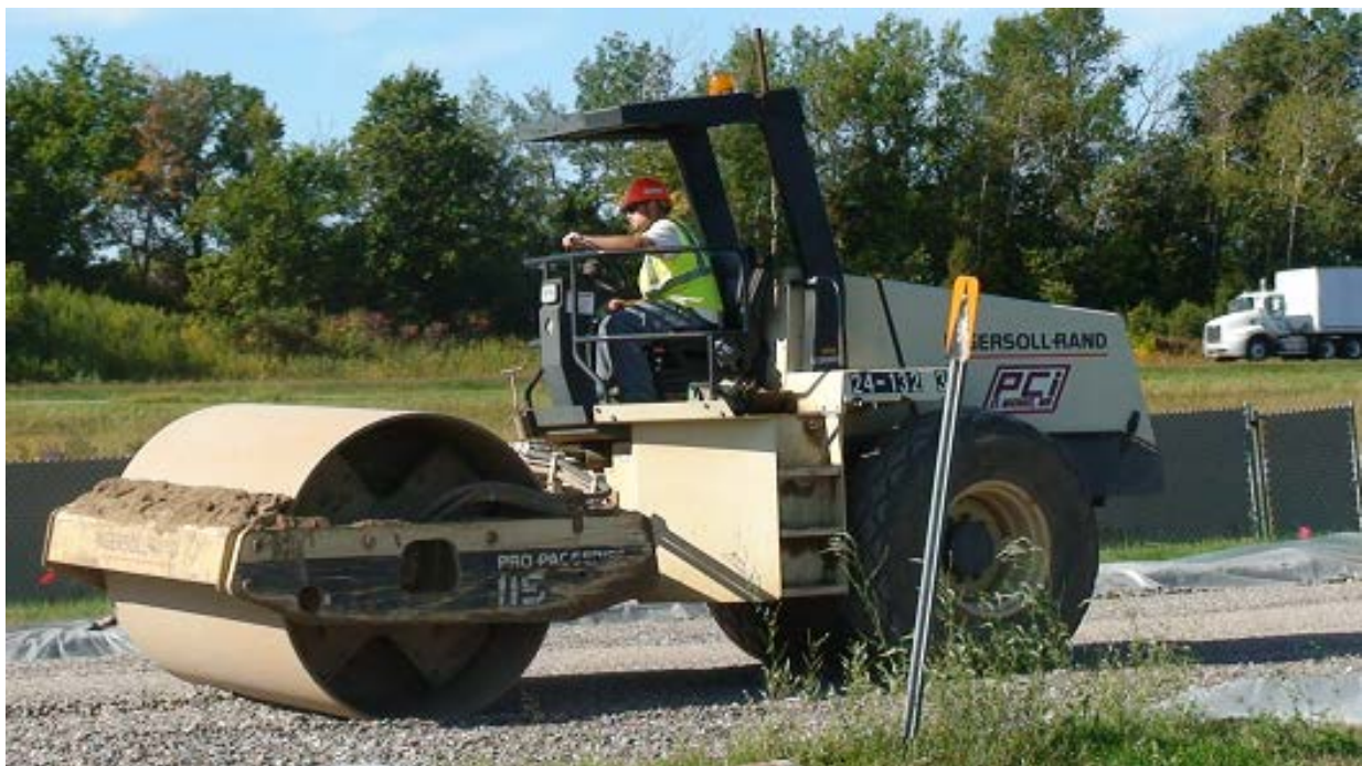
Figure 4.4. Placement of CA-15 base material
