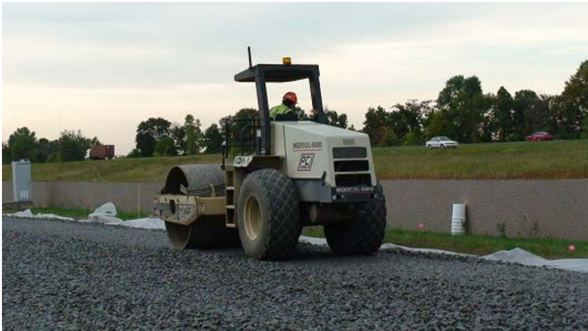
Figure 4.6. Light rolling to seat base material
