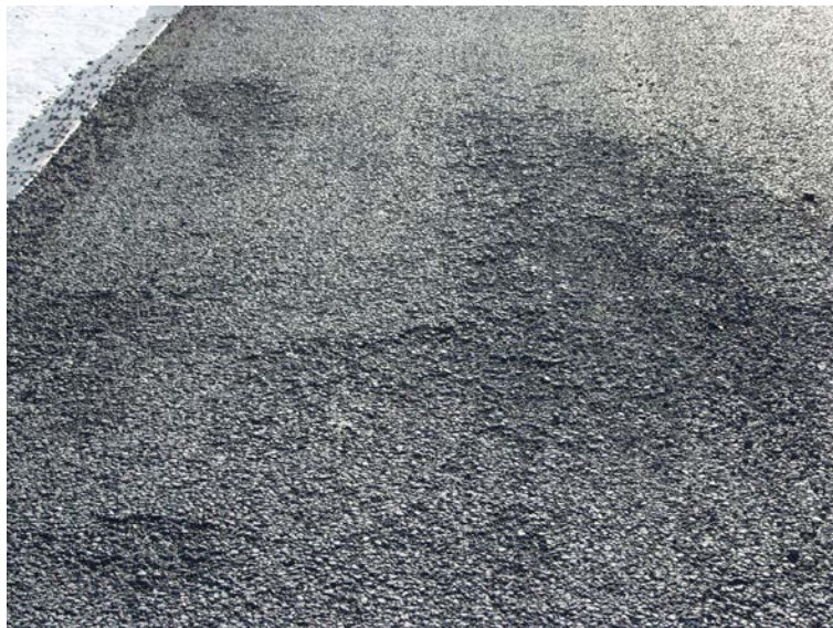
Figure 5.10. Surface raveling, cell 88
