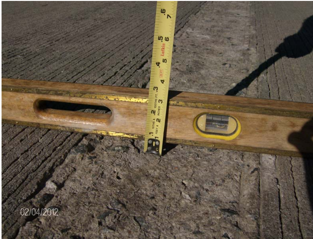
Figure A.3 - Wheel Path Spalling Depth
