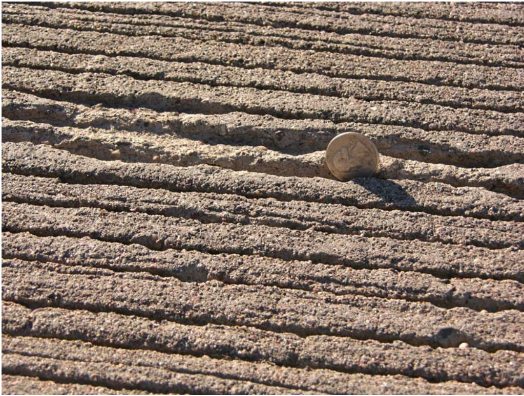
Figure A.5 - Early Stage Spalling
