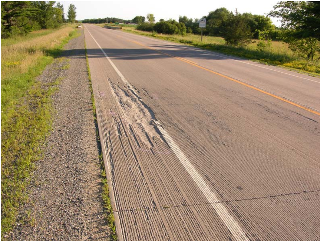
Figure A.4 - Shoulder Spalling
