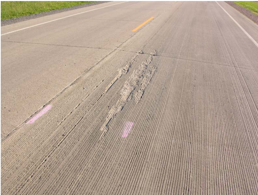
Figure A.6 - Wheel Path Spalling with Early Stage Spalling Surrounding It
