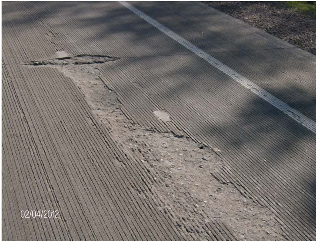
Figure A.1 – Wheel Path Spalling
