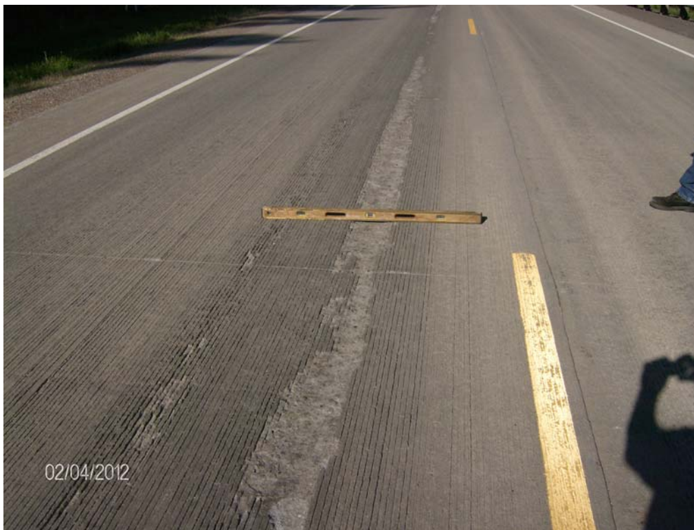
Figure A.2 – Wheel Path Spalling
