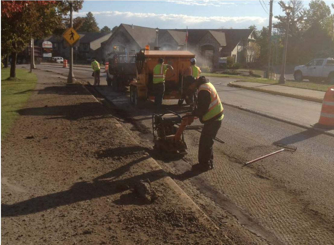
Figure 8. Patching Joint Cavities with HMA
