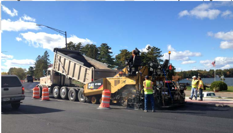
Figure 10. Paving Unit and Quad-Axle Dump Truck
