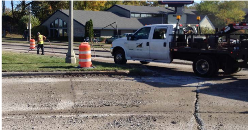
Figure 6. Air Lance Removing Debris/Deteriorated Concrete from Joint
