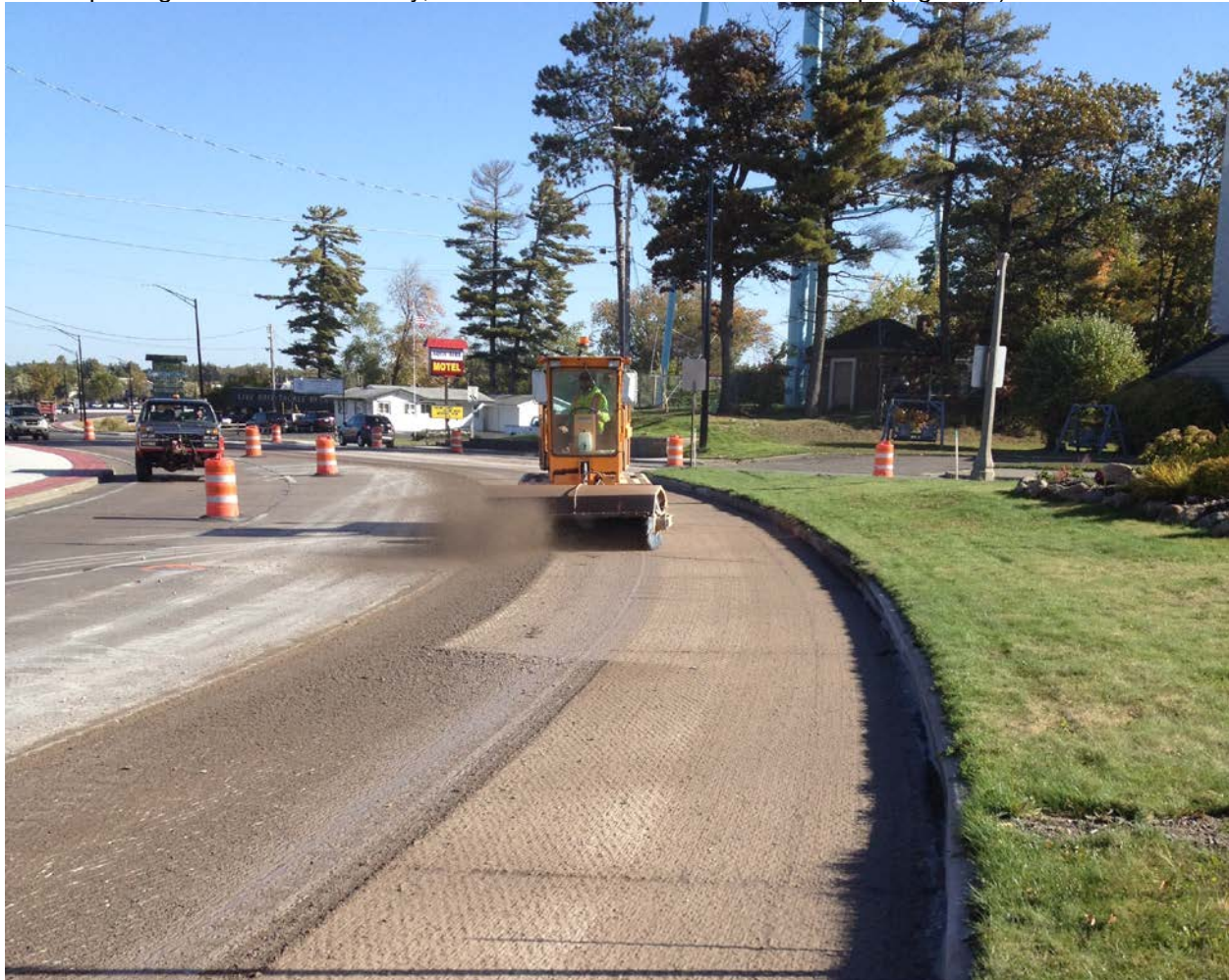
Figure 5. Sweeping Mill Tailings from Pavement
