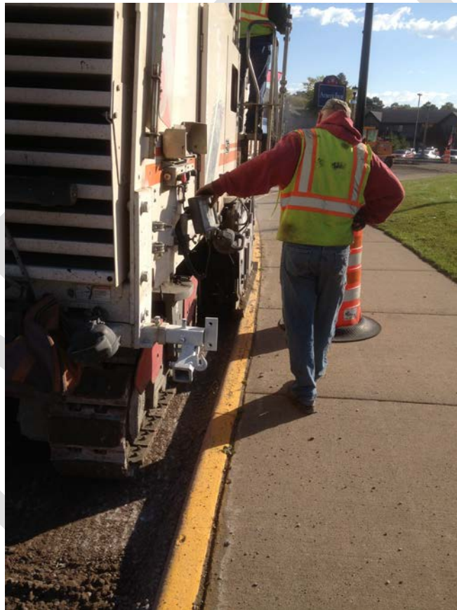
Figure 2. Large Mill Removing Tight to Curb Face
