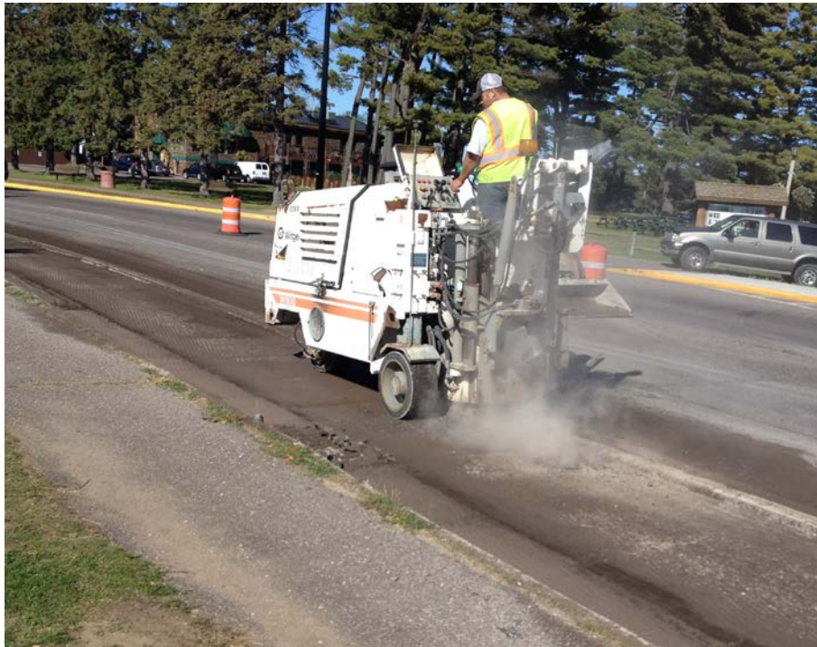
Figure 3. Small Mill Removing Concrete Around Structure
