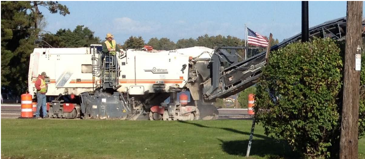
Figure 1. Large Mill Removing Mainline Concrete
