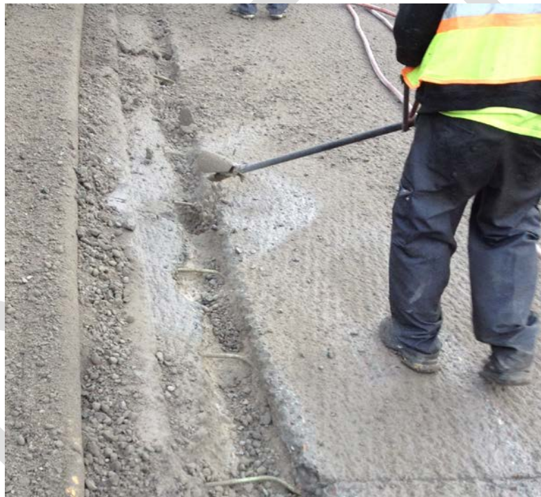
Figure 7. Air Lance Removing Debris/Deteriorated Concrete from Joint
