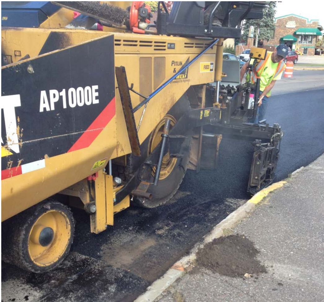
Figure 11. Paving Unit Approaching Project Butt Joint
