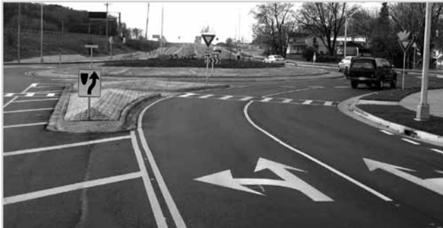
Figure 2.11a: WIS30 and Thompson Drive in Madison
